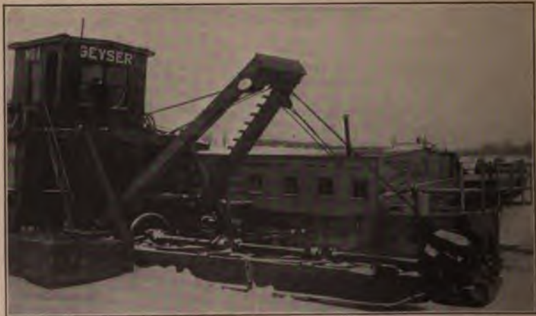
Cutter and Suction Pipe of Hydraulic Dredge.
